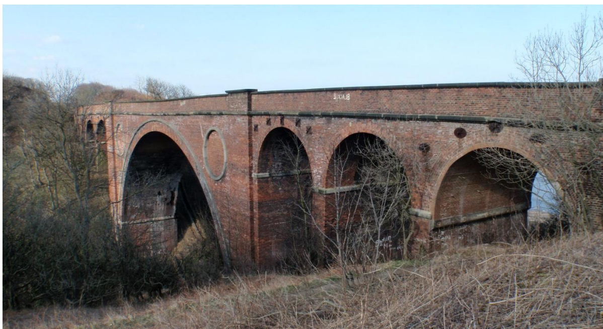
LEN3/229 Hawthorne viaduct
